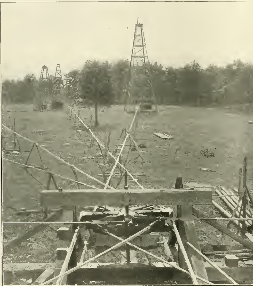
TRANSMISSION MECHANISM USED IN PUMPING.
